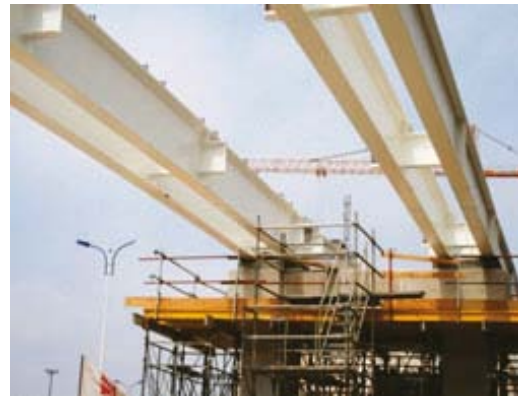
Fig. 20: Hoisting of preassembled pair of girders and subsequent welding of I-cross-beams to the prefabricated support stub
