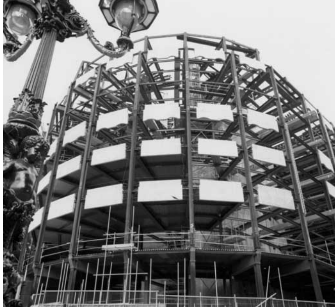
Bild 1a (links): Grand Buildings Trafalgar Square/ London (Montage)
