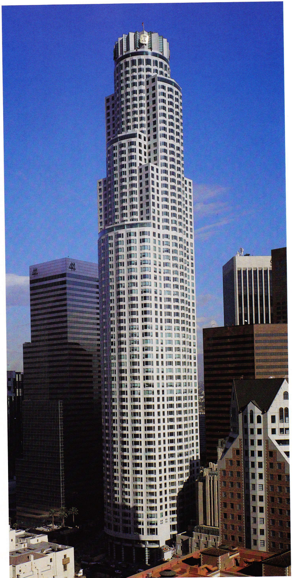
First Interstate World Center, Los Angeles
