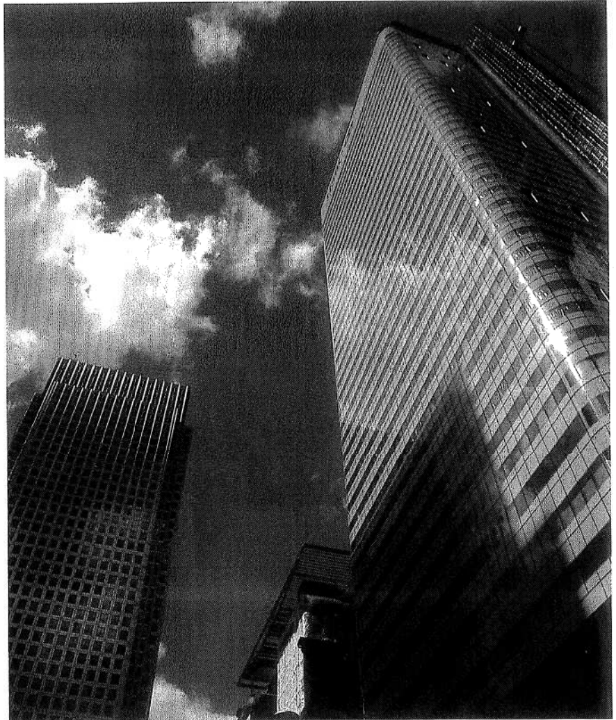
London Docklands. Canary Wharf, HSBC Headquarters (rechts)
