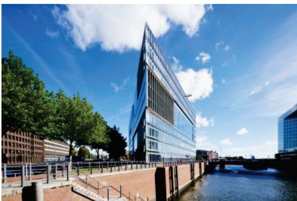
Fig. 2: The ten-storey building “Deichtor-Center“ in Hamburg Hafencity is protected by a R30 fire protection coating.
