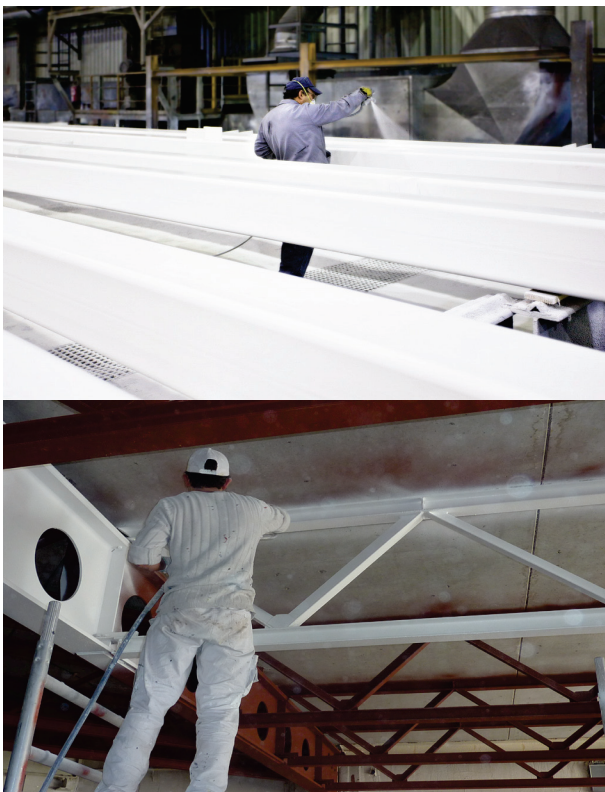
Fig. 14: The airless spraying method ensures fast, even and economical coating. It can be used both off site and on site.
