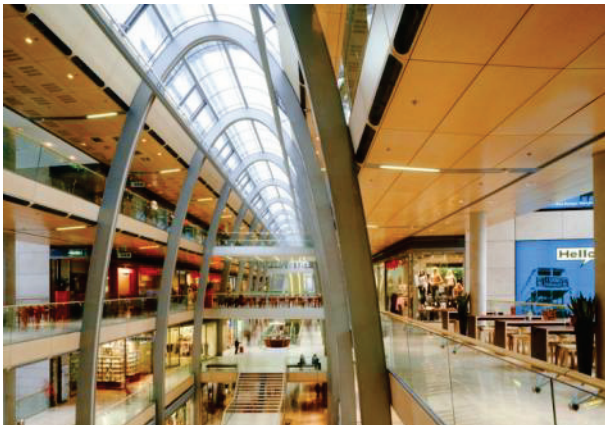
Fig. 11: The 30,000 m 2 of the “Europa Passage” in Hamburg completed in 2009 can accommodate 120 shops and businesses. Office space is located above the passage. The passage’s striking steel structure is protected by an R90 solvent-based fire protection coating.
