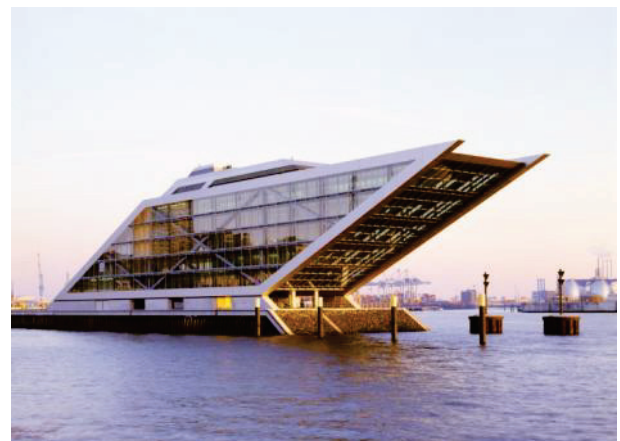
Fig. 9: The office building “Dockland” in the port of Hamburg, protected by an R30 fire protection coating, projects out in the form of a parallelogram over the water like the bow of a ship.
