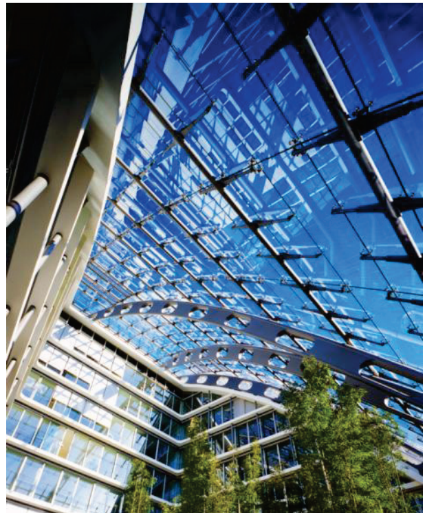
Fig. 1: A water-based fire protection coating protects the steel structure of the “Berliner Bogen”, an eight-storey office building with 43,000 m 2 gross floor space completed in 2001.
