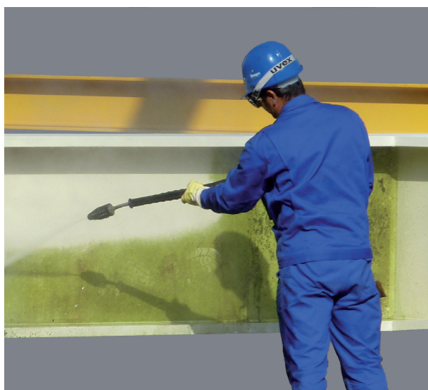
Fig. 16: Contaminated fire protection coatings can be cleaned by blowing, vacuuming or lightly brushing the dirt off. Some coatings can even be cleaned with high-pressure cleaners.
